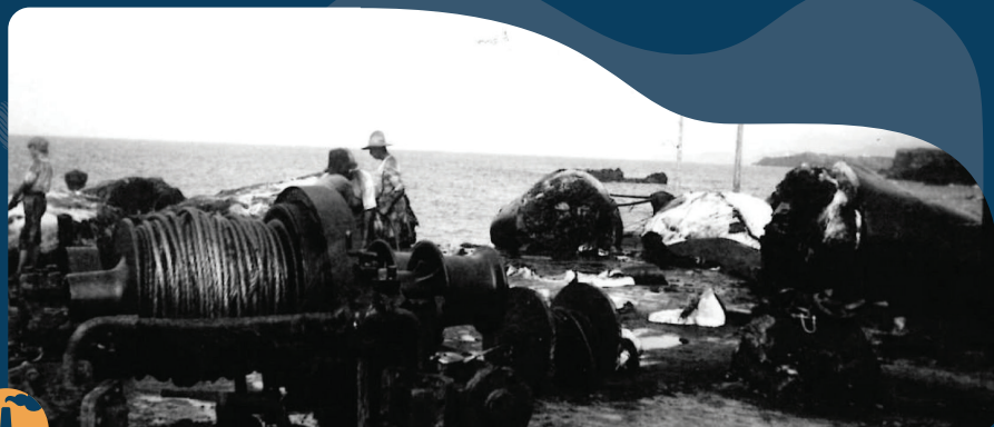
Antigo guincho que puxava as baleias para terra, para posterior desmanche. Old winch used to pull the whales to land for subsequent processing.
